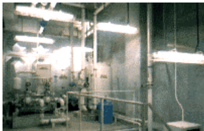
Aichi Prefectural Library's facilities for use of rainwater(pump room & water collection tank)
